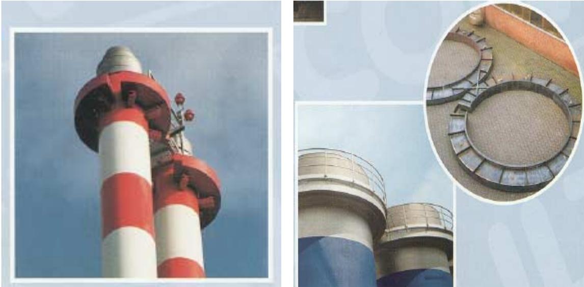
**Figure 1.10 TLDs installed in chimneys**
