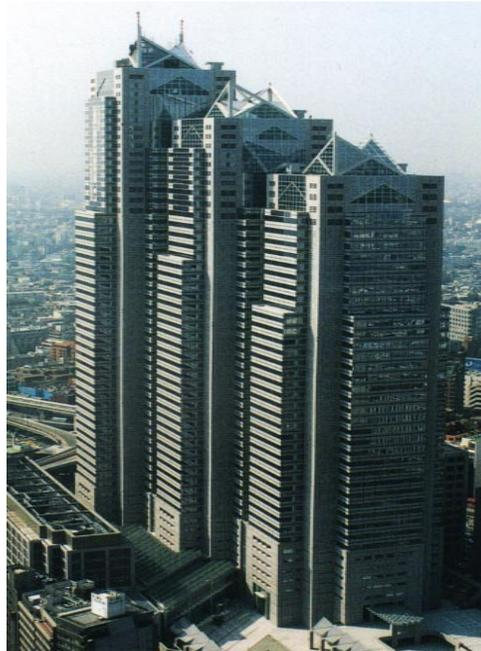
**Figure 1.1(b)** Shinjuku Tower using HMD
