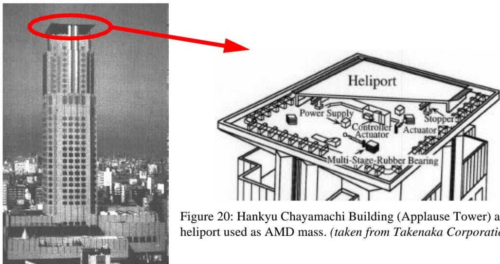
Figure 20: Hankyu Chayamachi Building (Applause Tower) and heliport used as AMD mass. (taken from Takenaka Corporation)
