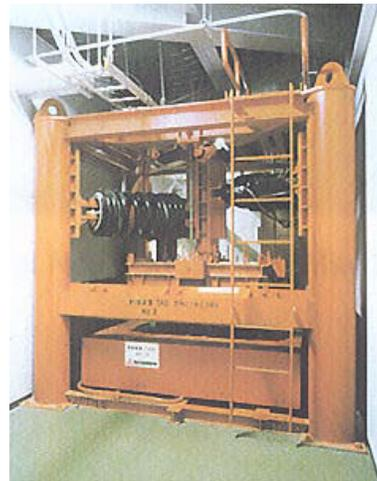
Figure 28. Kansai International Airport Tower and HMD unit installed within.
