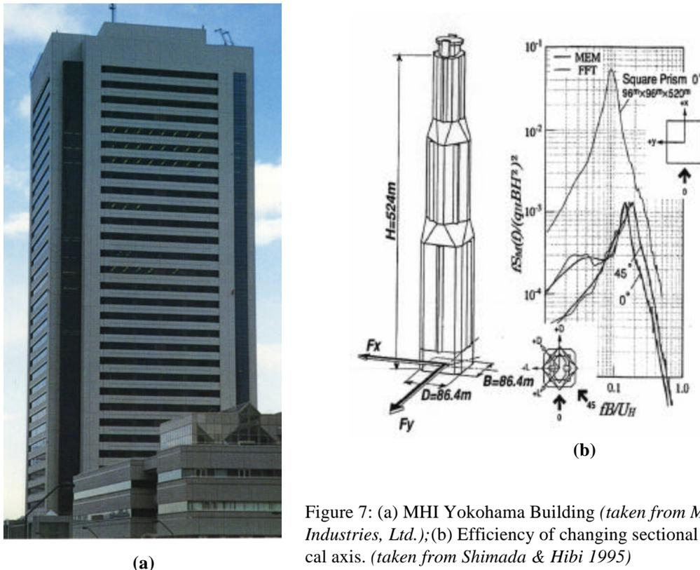
Figure 7: (a) MHI Yokohama Building (taken from Mitsubishi Heavy Industries, Ltd.); (b) Efficiency of changing sectional shape along vertical axis. (taken from Shimada & Hibi 1995)
