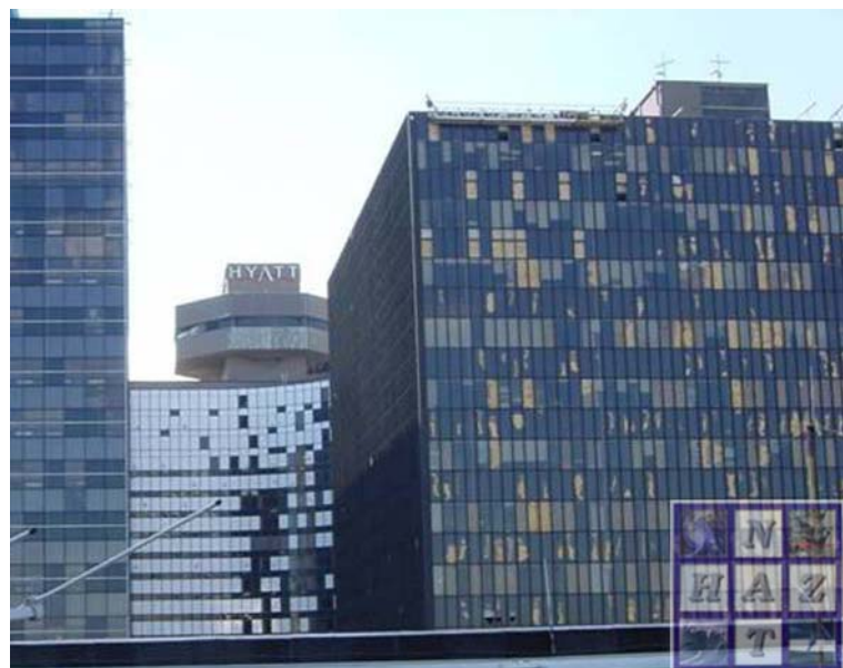
Figure 2 Damage to Hyatt Regency Hotel and Amoco Building as seen from the roof of City Hall
