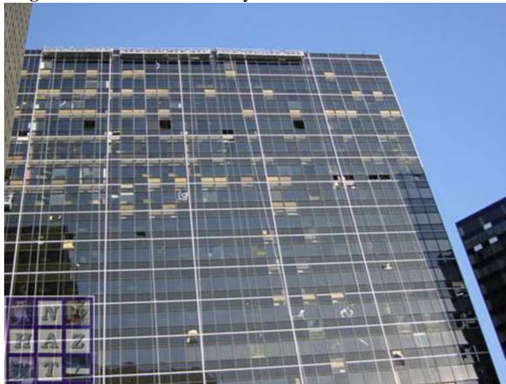
Figure 6 West face of 1250 Poydras.
